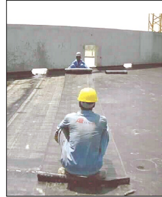
Laying Uniflame APP Membrane
